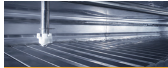
Clean-in-Place (CIP) Upgrade for Existing Freezers
